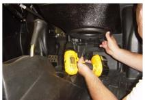
Screw the speaker in tightly ands seal any holes NOTE: Sealing holes to prevent air leaking will improve sound quality,
